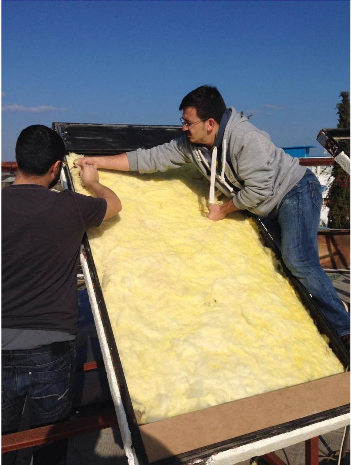
FigureA5 : Fitting glass wool in collector
